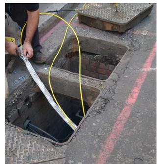
Figure 13: Cable being deployed in existing duct infrastructure in a harsh environment
